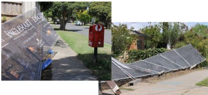
Photos: Recent examples of collapsed Temporary fencing with shade cloth attached upturned during strong wind gusts
